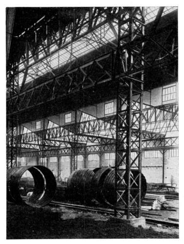
$\label{eq:Fig. 2.} Factory building 70 m <math display="inline">\times$  40 m at Pont-Ste-Maxence.
