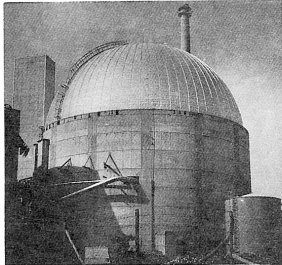
Fig.4 Completed reactor with aluminium cladding
