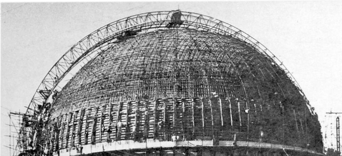
Fig.2 Mobile scaffolding for hemispherical dome
