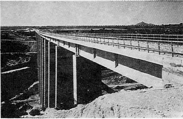
Fig.29 Bridge on Oran-Benisaf line, Algeria
