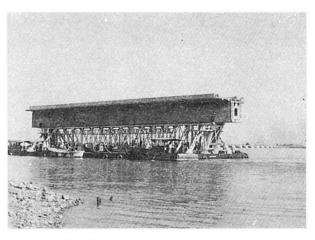
Fig.2 Girder being transported on a pontoon
