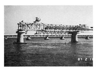
Fig. 3 Assembly of Segment
