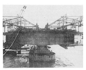
Fig. 2 Superstructure under construction
