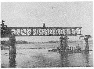
Fig. 4 Movement of Assembly Truss
