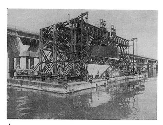
Fig. 1 Floating Gantry with Cofferdam Assembly
