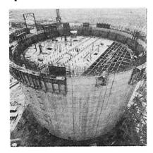
Fig. 2 Containment under Construction
