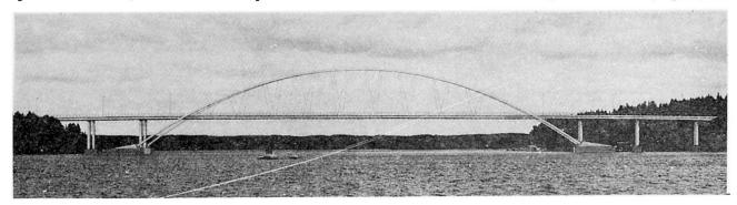
Fig. 4. A proposal for the application of a steel-concrete composite arch.
