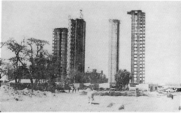
Fig.10 Slipformed Lift Cores
