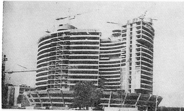
**Fig.10 Slipformed Lift Cores**
