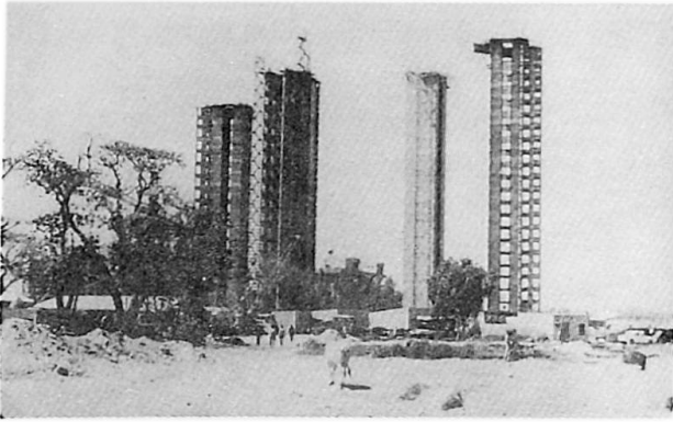
Fig.10 Slipformed Lift Cores
