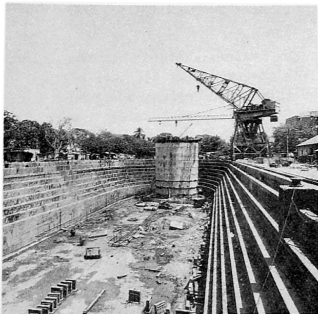
Fig.1 Caissons precast in dry dock
