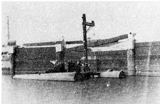
Photo.5 Launching camel placing RC planks
