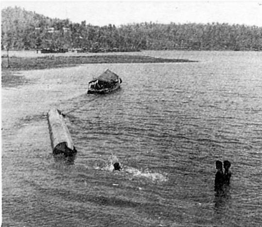
Photo.3 1000mm diameter casing being towed to site
