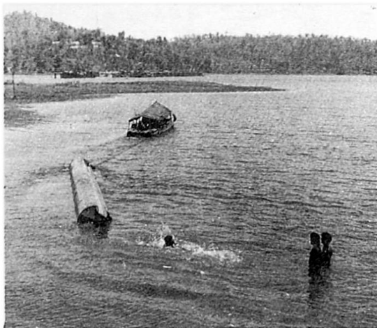
Photo.3 1000mm diameter casing being towed to site
