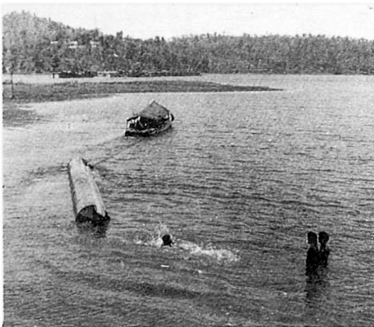
Photo.3 1000mm diameter casing being towed to site
