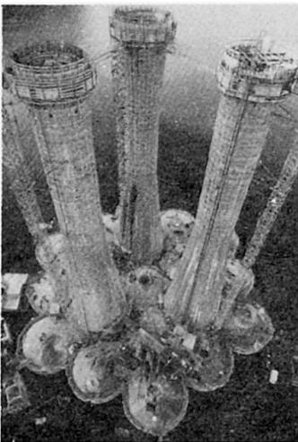
**Fig. 5** Platform TCP2 under construction in Norwegian Shipyard
