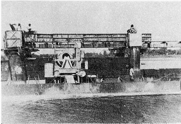
Photo 6 Concreting of cast in situ longitudinal bracings.
