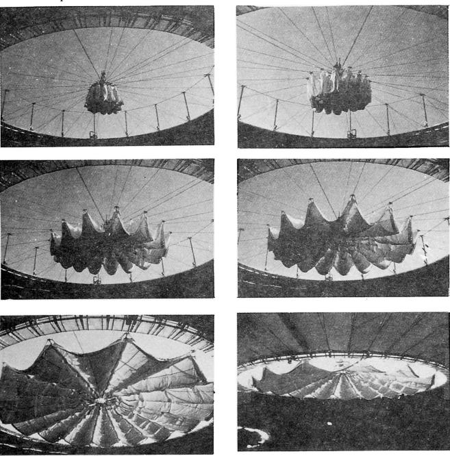
Fig. 15 Arena Zaragoza Opening/closing procedure of the 1 000 m² inner membrane roof.
