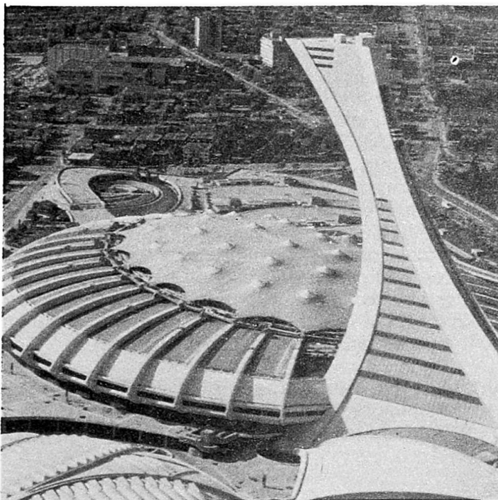
Fig. 7 Olympic Stadium Montreal Membrane roof area: 20 000 m 2 ; suspended from a 170 m high tower.
