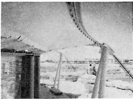
Fig 4.1 Eye Loops, Boundary or Ridge Cables on Masts
