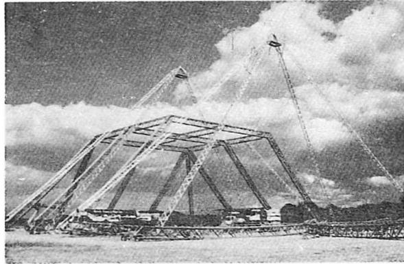
Figure 2 - Framework during erection
