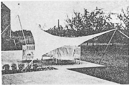
Fig 2.3 Minimum Surface Bounded by 4 Cables and 2 Masts
