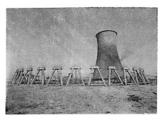
Fig.3 Precast diagonal column systems under erection
