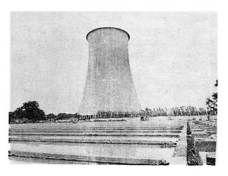
Fig.2 An NDCT with a lath casting yard in the foreground.
