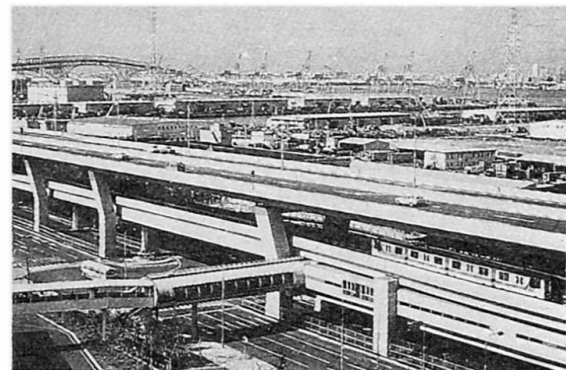
Fig. 9 Modern expressway/trunk combination: Osaka - Wangan Route
