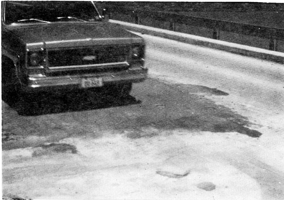
Fig.4 Bridge deck repaired by polymer concrete
