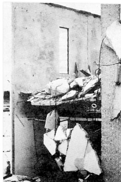
The tilt-up prestressed walls and the cast-in-situ post-tensioned beams were correctly proportioned in terms of section-by-section analyses. No thought or attention was given to tieing the various members together. The beams had no supports under their ends and were rubbing by friction on the walls -- when friction was broken, the building collapsed.
