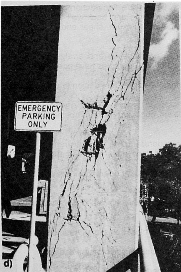
Fig 3. Bridge Damage, Loma Prieta 1989 (M7.1)
