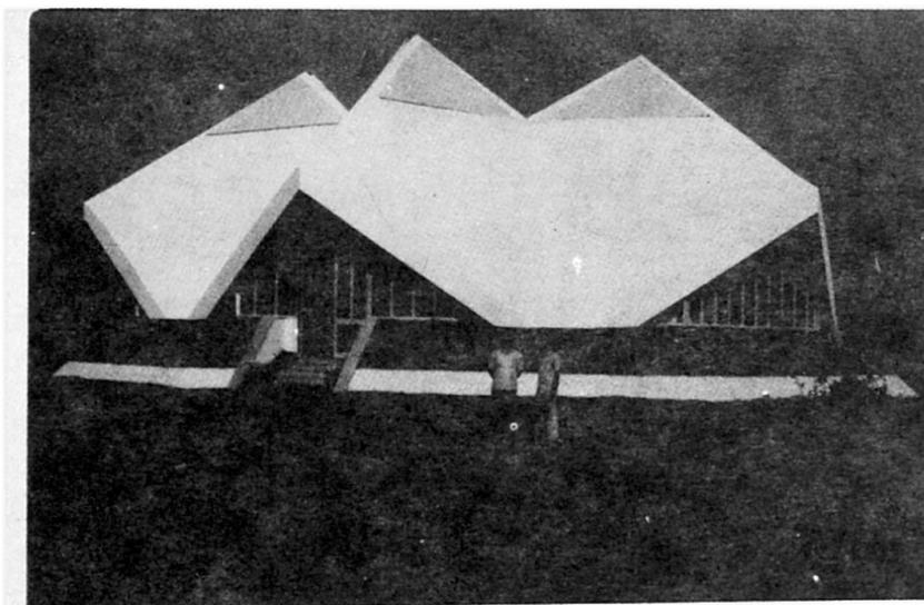
The topmost point of these intersecting hollow cubes shaped roof is at six meters above hall floor level as seen in Fig.2 & 3. The slopes of roof panels and supporting edge beams are of the order of  $55^\circ$ . A cutout on top of each cube provide ingress of natural daylight.
