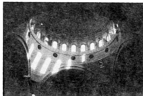
Structural connection between pendentive and main dome is to be done by supporting the dome in four position by means of hydraulic jacks capable to produce force of 3000 kN each (total force 12000 kN). These means that pendentive will take care of additional loads coming latter from applied mortar, mosaic and outside marble.
