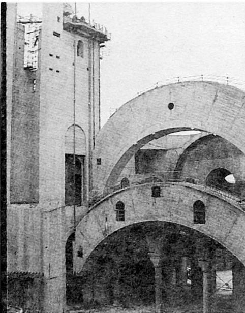
which belong to the wing sections, the semi-domes have been formed, each consisting of eight curved reinforced concrete trusses covered with curved slab decking.
