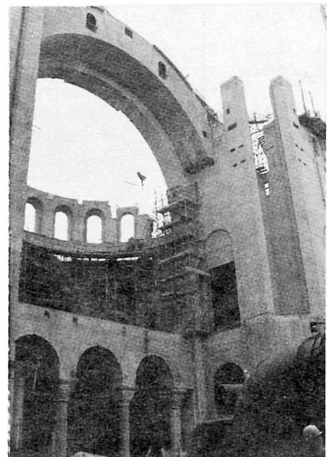
foundations, the existing part and the new structure of the forthcoming stages of construction was achieved with reinforced concrete columns and tie-beams.
