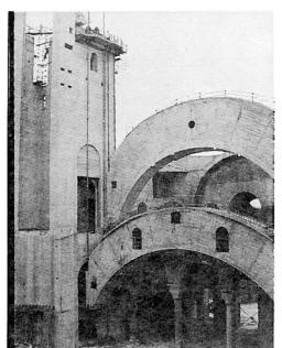
which belong to the wing sections, the semi-domes have been formed, each consisting of eight curved reinforced concrete trusses covered with curved slab decking.
