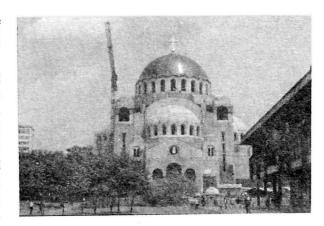
All arched shapes of the galleries and vaults have been transformed into assemblies of elements curved in two dimensions which, having been erected, form a three-dimensional shape. The semi-domes and the dome have been linearized by designing a system of arched trusses and two layers of curved decking. The precast parts are bound into a whole by in-situ cast parts of the structure which provide the required safety and long life of the building.
