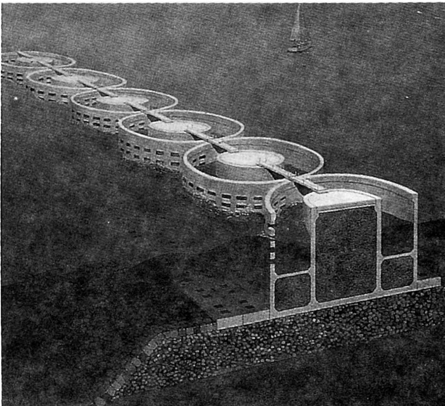
**Fig.7** Double-cylinder caisson-type breakwater
