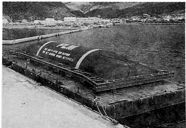
**Fig.4** Flexible-mound during airtightness test on a barge (40m(L) x 9m(W) x 3m(H))
