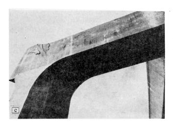
FIG 5. Earthquake Damage, Loma Prieta 89, China Basin Viaduct
