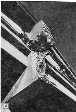
FIG 1. Bridge Damage During the 1989 Loma Prieta Earthquake
