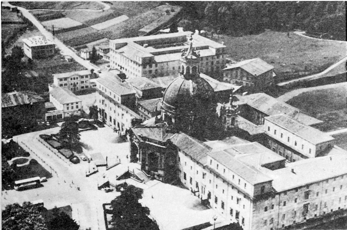
Pic.25: Basilica of St. Ignatio de Loyola in Spain
