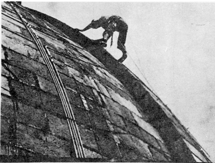
Pic.33: The operations to place the cables
