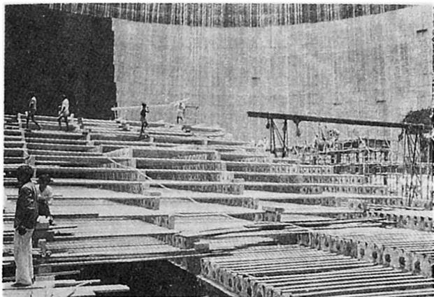
Fig.5 Assembly of laths for the packing in progress
