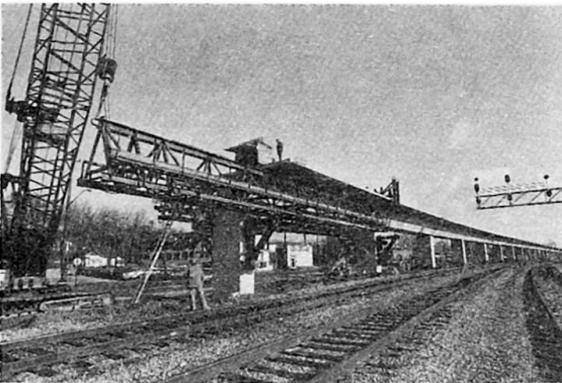
Fig 5. Segmental Construction of the Atlanta Transit System
