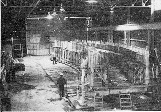
Fig. 4 Adjustable Form for Box Girder Beam Fabrication
