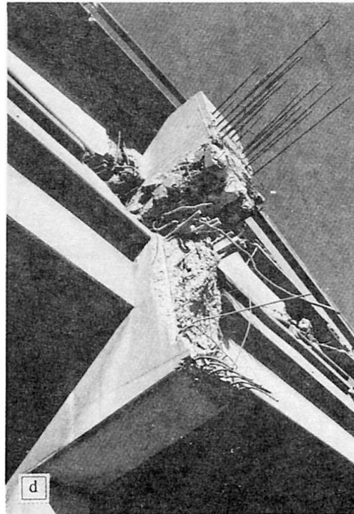
**FIG 1. Bridge Damage During the 1989 Loma Prieta Earthquake**
