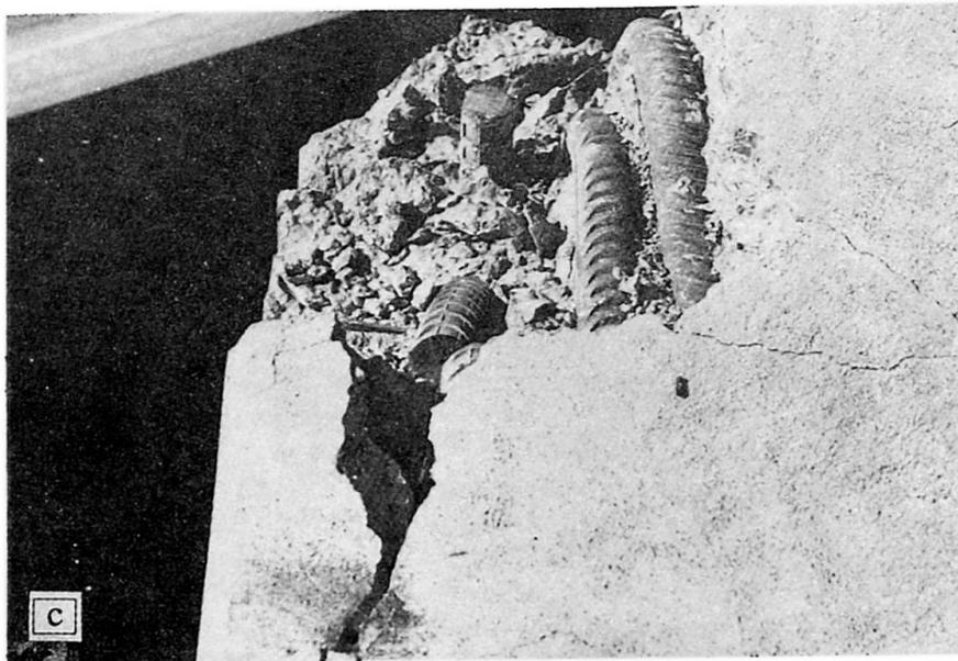
**FIG 9. I-980 Oakland, CA, Encountered Damage Patterns**
