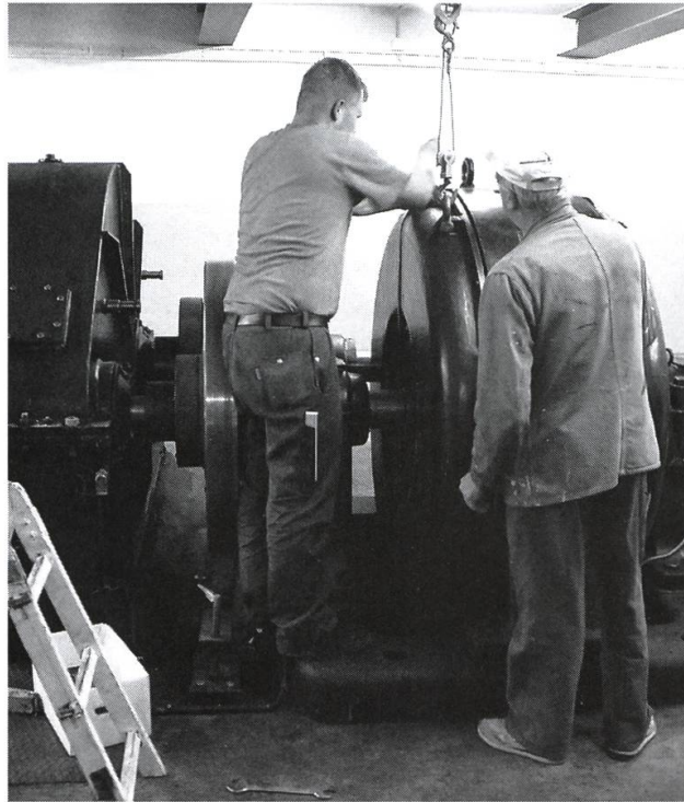
Renovation des Generators.
