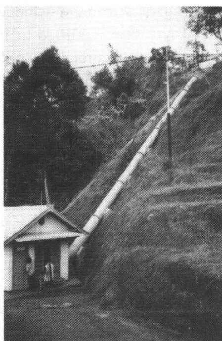
Figure 2: Medium-head Mini Hydro in Cicemet, Indonesia 4
