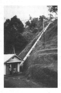
Figure 2: Medium-head Mini Hydro in Cicemet, Indonesia<sup>4</sup>
