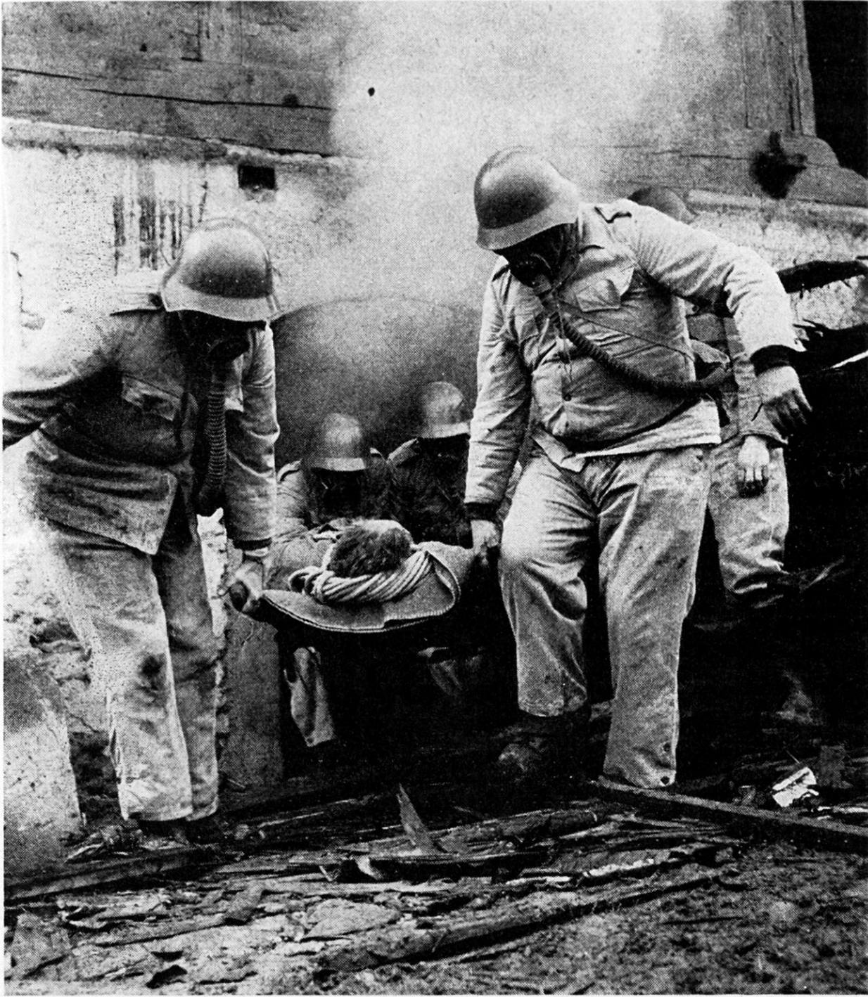
Photo W. Nydegger
