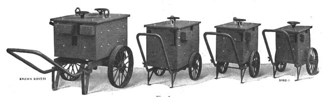
${\bf Fig.~3.} \\ {\bf Brown\text{-}Boveri\text{-}Schweisstransformatoren}$
