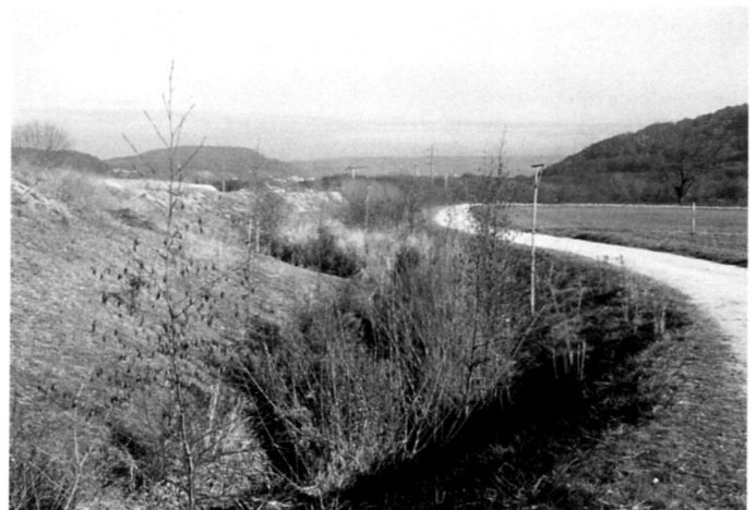
Left: Suspended grid to secure an embankment.
