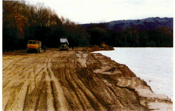
Shore before and during rubble filling.
