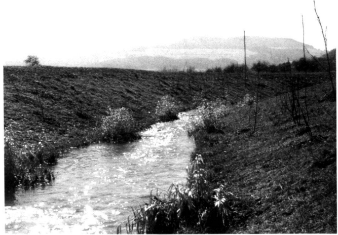
Left: Embankment protection with fascine, open fascine layer combinations (1 year after planting).
