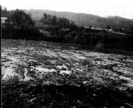
Subsequent creation of a basin in an extensive filled-in area to collect surface water; the overflow is designed as a wide "track" feeding into a filter system so that no fine particles can be washed into the lower lying spawning areas. Formation of a mowed area along the side which is delineated on the inner side by an earth bank which has still to be planted.
