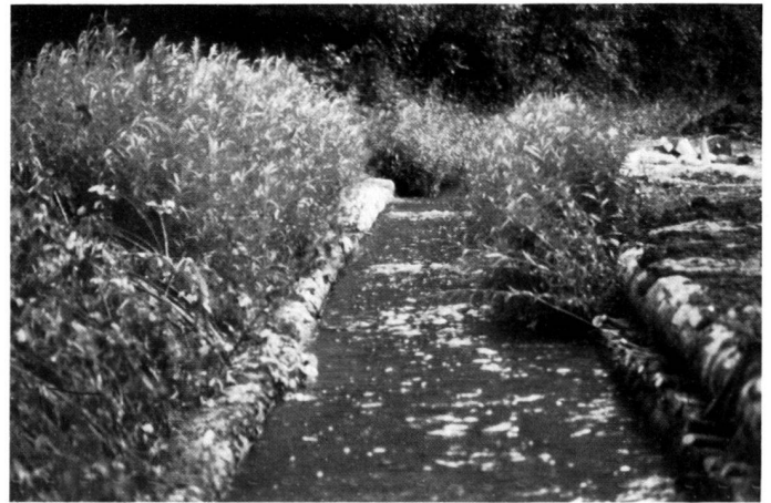
5 Left, layer of leaf blade with pine trunks to secure the base; right, 2 pine trunks with a layer of bush in between.
