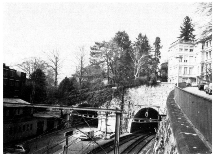
Left: Existing old stone wall near Falkenburg/Hohenbühl with west entrance to tunnel.
