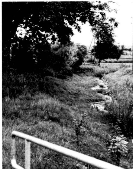
The course of the stream to the east of the Wilenhof bridge shows that, where possible, the existing stocks of trees and bushes were retained during construction and how, on the left-hand side, the surviving reeds are able to spread once more on the extremely flat embankment. Picture 1 was taken in March, picture 2 in June and picture 3 in August 1982.
