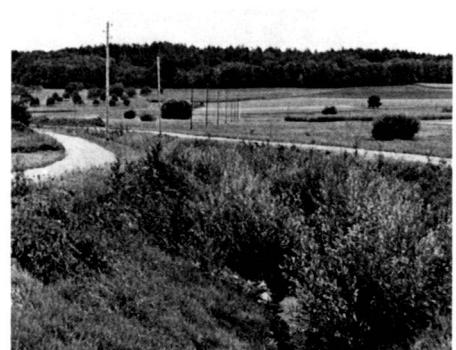
The pictures show the course of the brook to the west of the Wilenholz bridge with varying widths of channel and differing embankment gradients. Picture 1 was taken in March, picture 2 in June and picture 3 in August 1982. The sequence shows how quickly the willow bundles sprouted and grew and how the greenery was quick to spread on the embankments (no humus used) thanks to use of the appropriate seed mixture.
