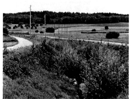
The pictures show the course of the brook to the west of the Wilenhof bridge with varying widths of channel and differing embankment gradients. Picture 1 was taken in March, picture 2 in June and picture 3 in August 1982. The sequence shows how quickly the willow bundles sprouted and grew and how the greenery was quick to spread on the embankments (no humus used) thanks to use of the appropriate seed mixture. Fotos: P. Bolliger
