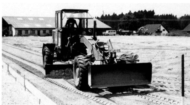
*Left:* Covering of surfaces with a nonwoven mat or filter sand, depending on the subsoil.
