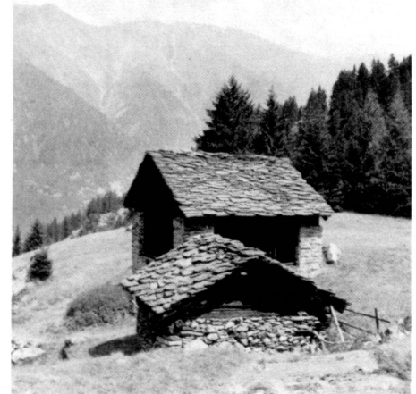
Above: Summer pasture dwelling near Stürvis, Stierva, Grisons. Left: Housing settlement whose form has been adapted to the landscape in the Valle Indemini, Ticino. Below: In Bergell, Grisons. Architecture in harmony with the landscape. Photos Werner Blaser
