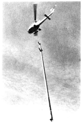
Transport eines 26-m-Mastes
