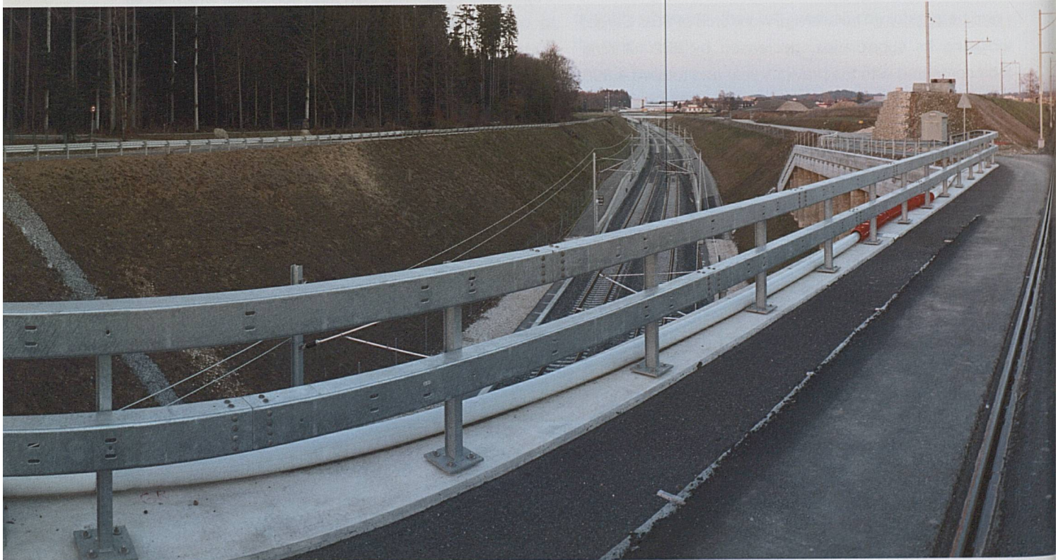
The new Rail 2000 route between Langenthal and Herzogenbuchsee
