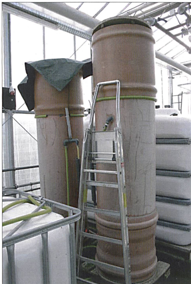
Fig.2: C. Slow rockwool filter (SRF).
