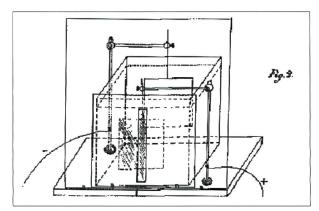
Fig. 4. Electrochemical actinometer wooden box (original engraving).
