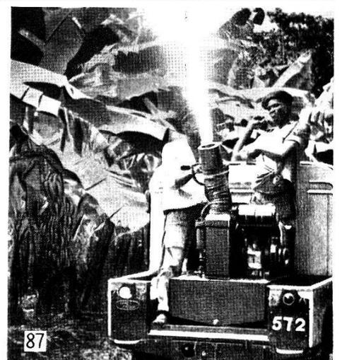
Fig. 79-87. Machinery for applying liquid insecticides.
