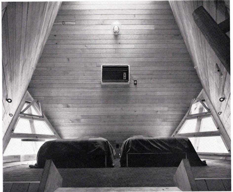
These cell units developed on the basis of stacked tetrahedrons were erected by the architects as early as 1968/69, and are among the first projects of this type ever realized. The leading advantages of this polyhedron design, aside from its static qualities, are its combinations and extension potentialities, as shown in the attached plan.
