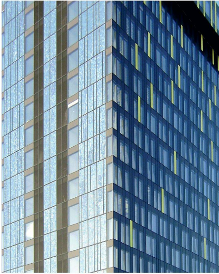
01 Power Tower, Linz (Foto: Sauter AG)
