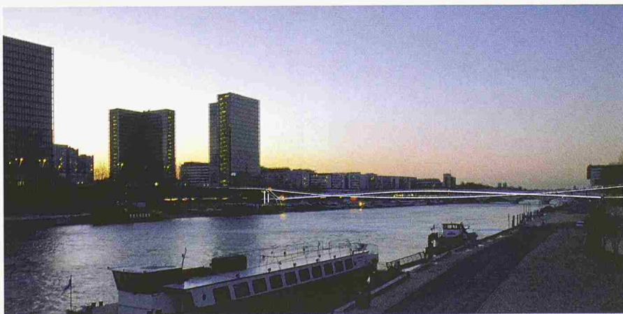
Passerelle at Bercy, Paris
