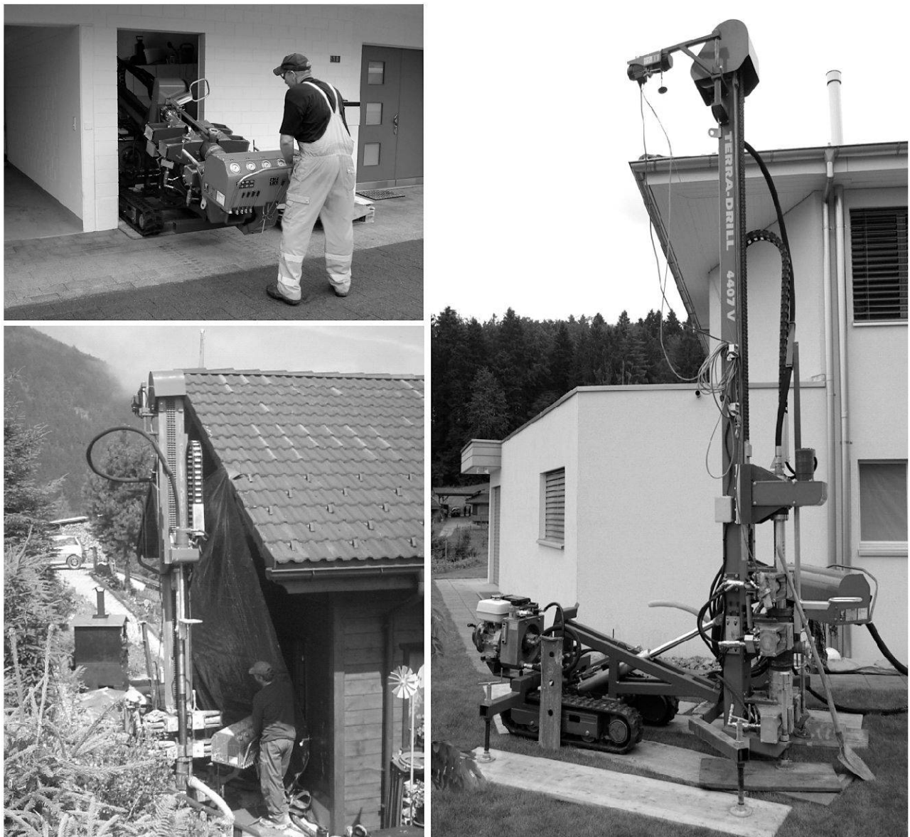
Fig. 5: Light and compact mini-rig to drill shallow (100–120 m deep) wells for deployment of geothermal heat pumps systems [source: Terra AG and J. Wettstein].
