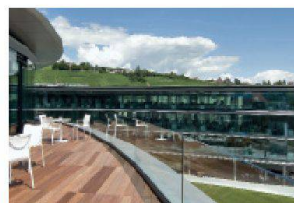
Swarovski Campus— main administration Ingenhoven architects international Düsseldorf, Männedorf Branch Männedorf
