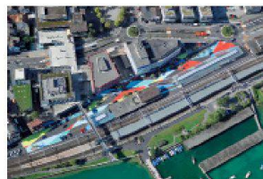
Reconstruction of railway station Horgen Hornberger Architekten Zurich
