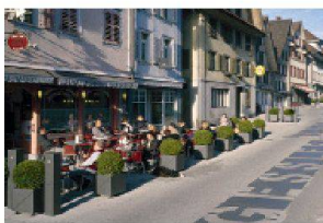
Revitalization of the Unterdorf part of Küsnacht hwp Architekten Hünenberg
