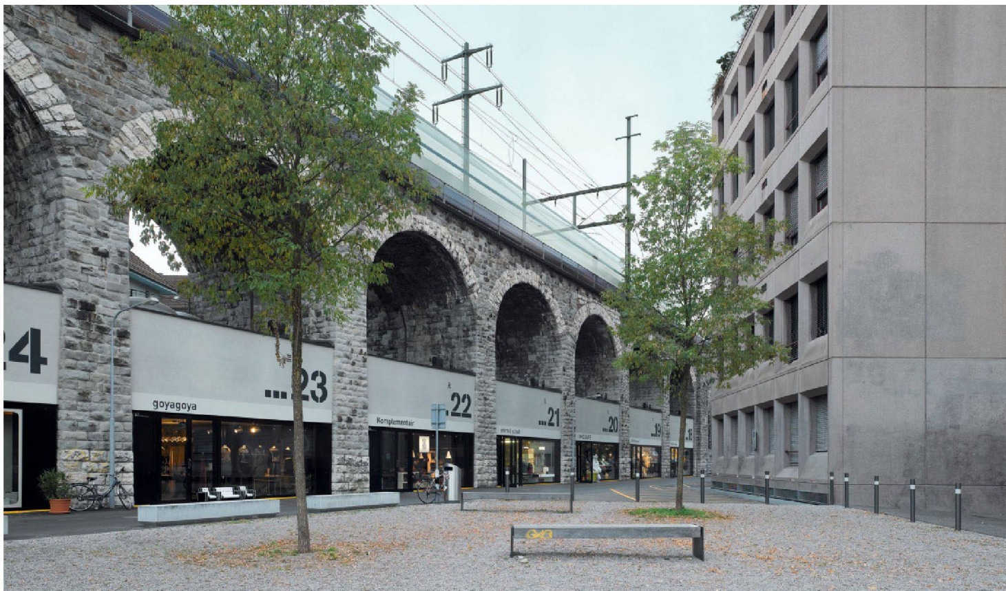
01 The former spatial barrier is now a unifying element (photo: Roger Frei)
