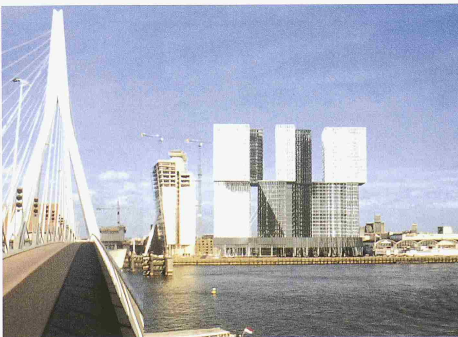
MAB Tower, Rotterdam, Netherlands
